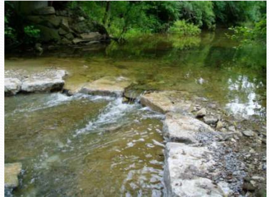
Upstream Pool Control, Mill Creek , Nolensville, Tennessee (after one growing season)
