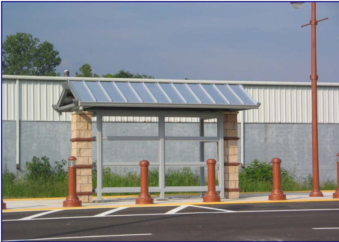
May 31, 2006 – Shelter at Mt. Juliet Station
