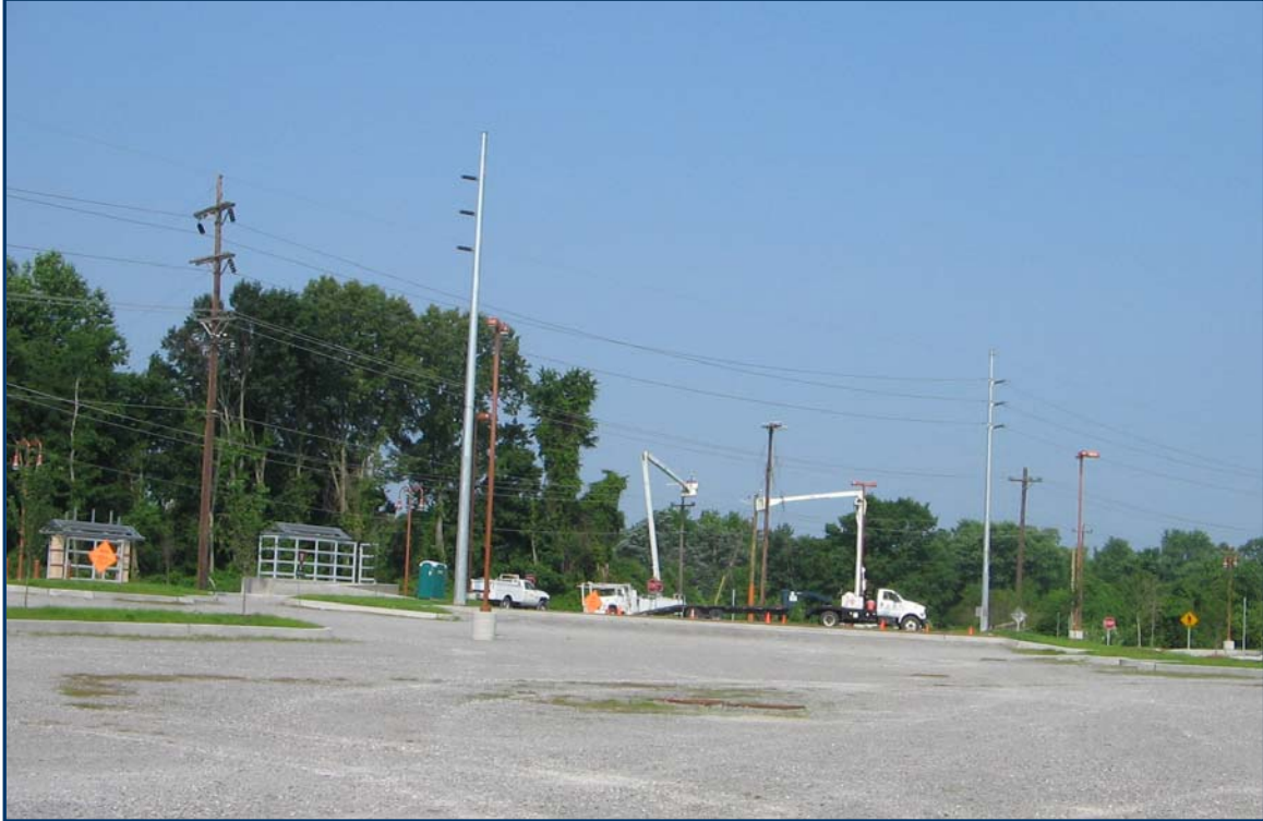
May 31, 2006 – Utility Relocation at Donelson Station
