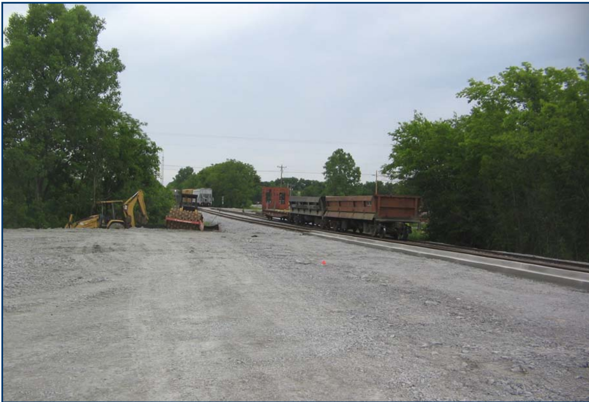
May 30, 2006 – Grading at Martha Station
