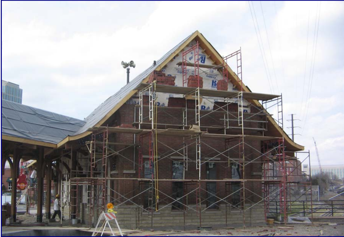
February 28, 2006 – Masonry Work at Riverfront Station
