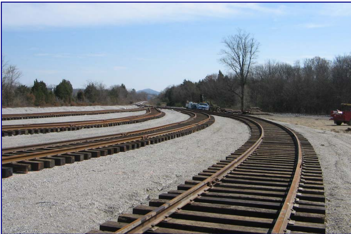
February 27, 2006 – Track Construction for the Lebanon Layover Facility
