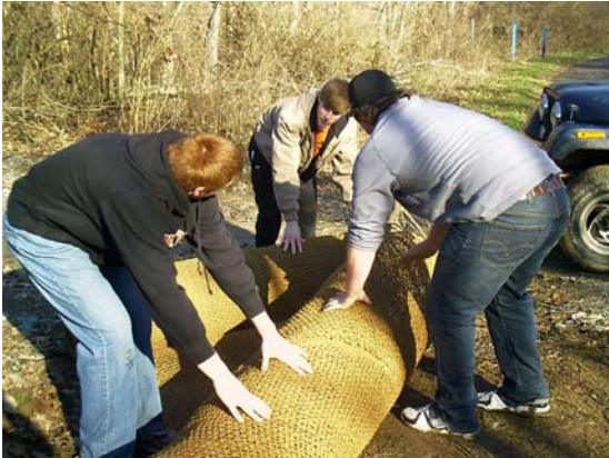
Students rolling the cedar trees in the coir matting and driving anchors into the bank above the revetments that were installed in December.
