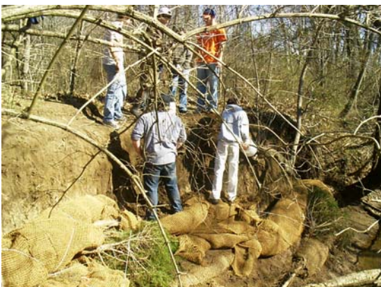
Cedar revetments are being lowered into place to be wired in, while other students plant trees in the upstream reforestation project area
