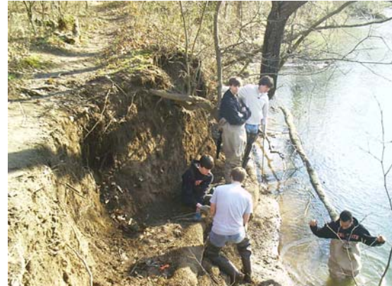
Students rolling the cedar trees in the coir matting and driving anchors into the bank above the revetments that were installed in December.
