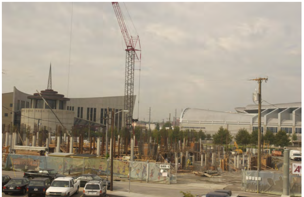
Schermerhorn Symphony Center under construction. Photograph, 2004: Courtesy of Vanderbilt University
