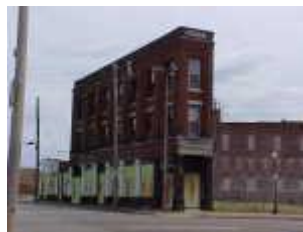
The Terminal Hotel in Chattanooga
