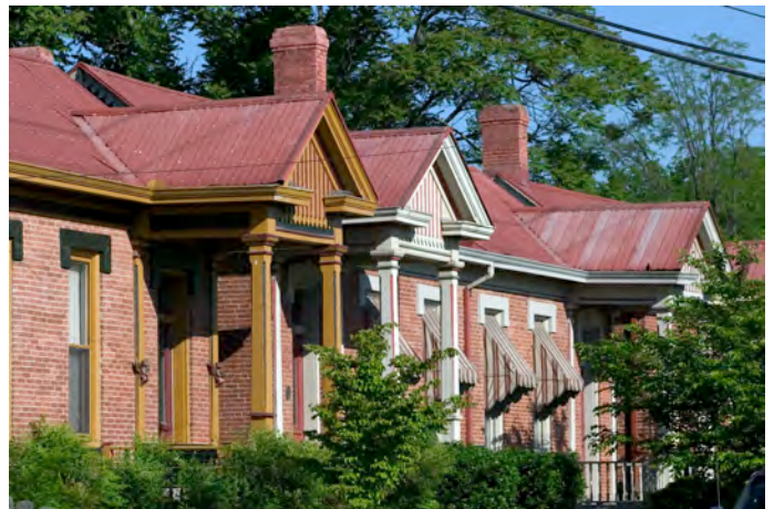
Above: Row houses on Fifth Avenue in the Germantown neighborhood define a consistent, human-scaled wall for the street. (photograph, 2005: Vanderbilt University, Neil Brake)
