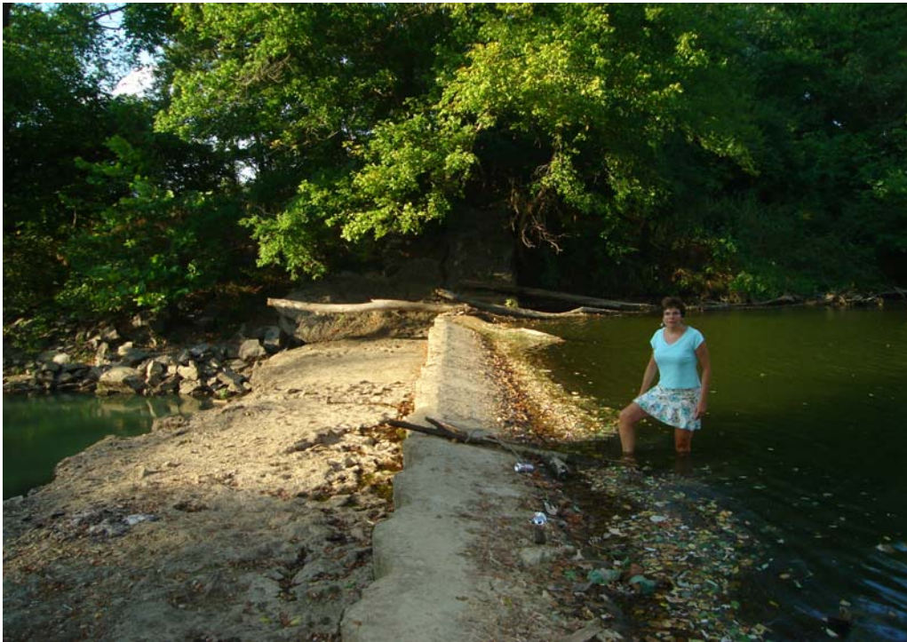
Low head dam, right foot on wall left foot on five plus feet of built up sediment behind dam. Visible lowering of water level behind dam between 1 and 5 pm.
