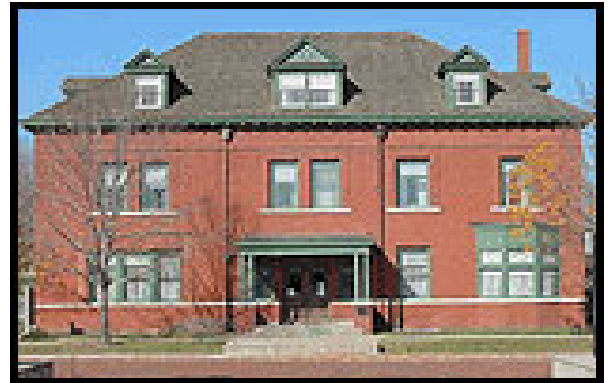
Durant-Dort Headquarters, Flint, MI
