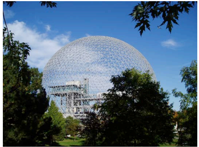
Figure 11. The Biosphère was once covered by a transparent acrylic skin. A fire destroyed this outer covering in 1976 and it was never replaced.
