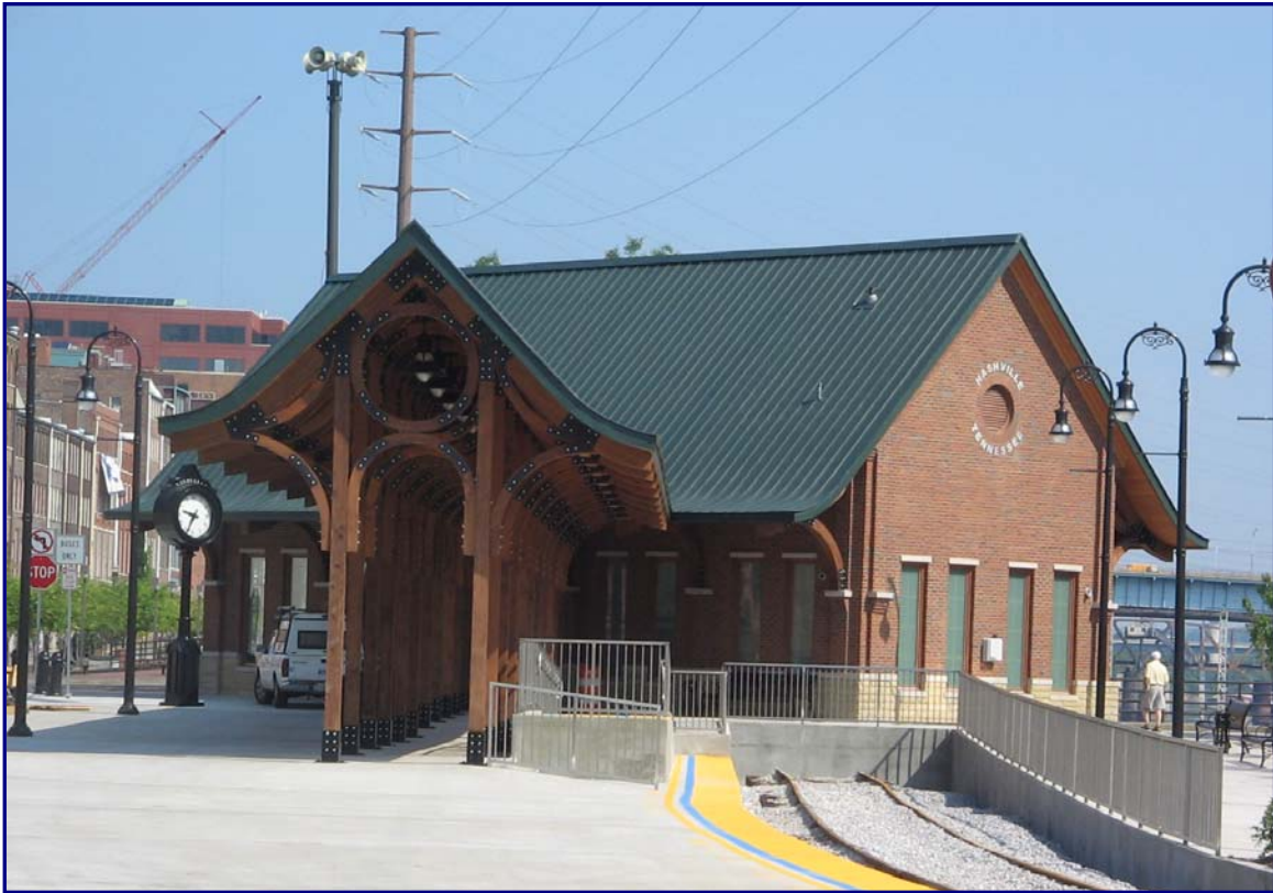
June 26, 2006 – Riverfront Station at Substantial Completion
