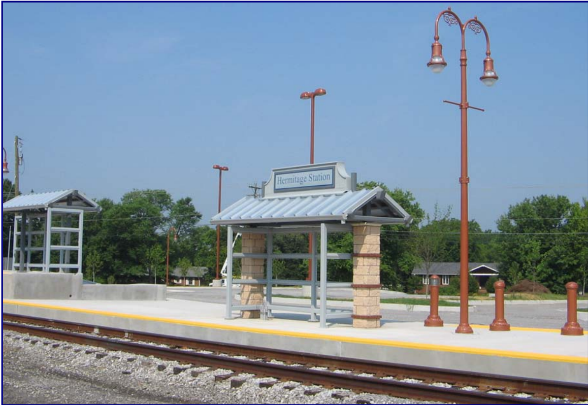
June 30, 2006 – Platform at the Hermitage Station
