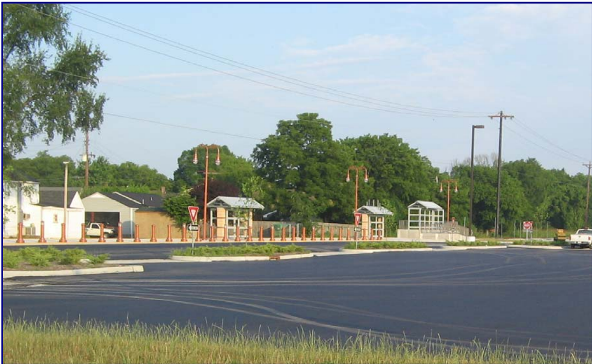
June 29, 2006 – Paving at Lebanon Station
