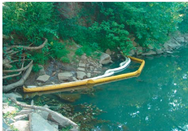
Absorbent booms are used to try to soak up chemicals that float on the surface.
