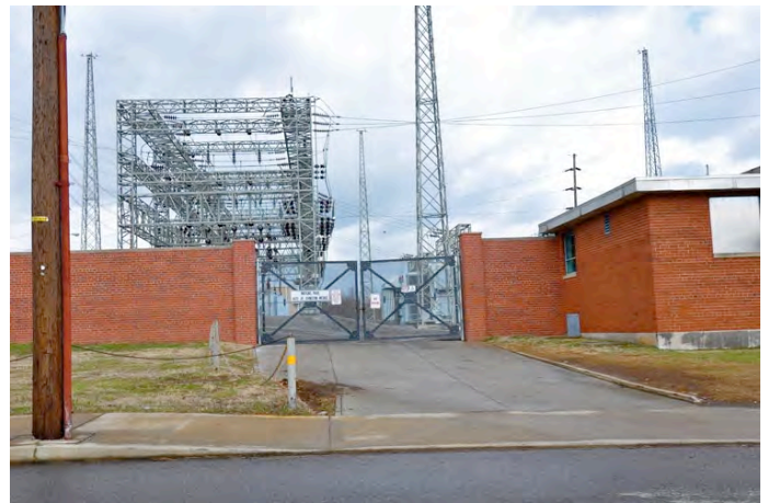
View of substation from Jo Johnston Avenue
