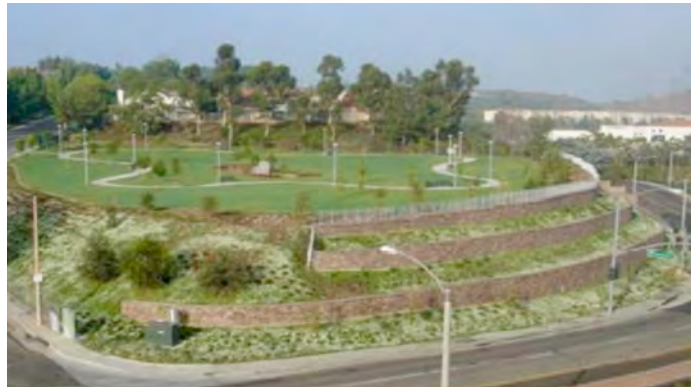
Roosevelt Park conceals substation enclosure
