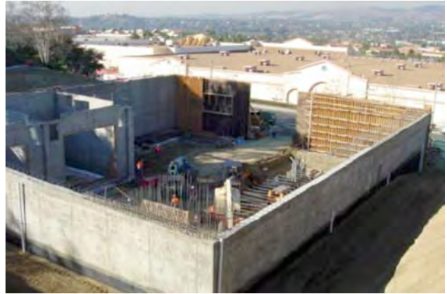
Construction of substation enclosure
