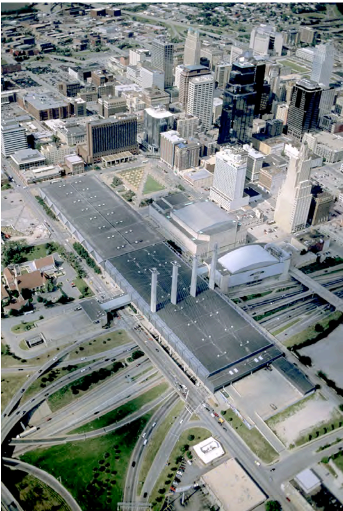
Kansas City's Bartle Hall Convention Center. Instead of shoehorning its expanded convention center into existing downtown blocks, Kansas City built the structure over the downtown interstate. The center, which is 330 feet wide, rises about 45 feet over the highway and two other downtown streets. Photograph, 2002: Alex S. MacLean/Landslides
