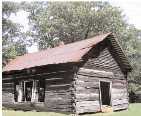
This rare postwar log schoolhouse is located in Henderson County.
